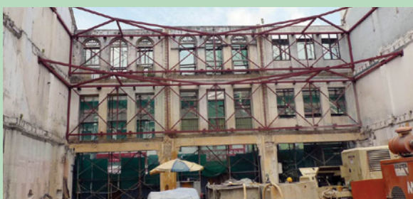
Front facade propped up using steel trusses
