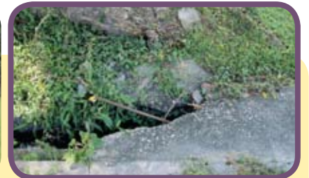
Broken drains
