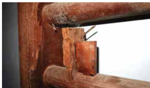
A hidden lock at the timber security grill; the wisdom of ancient carpentry
