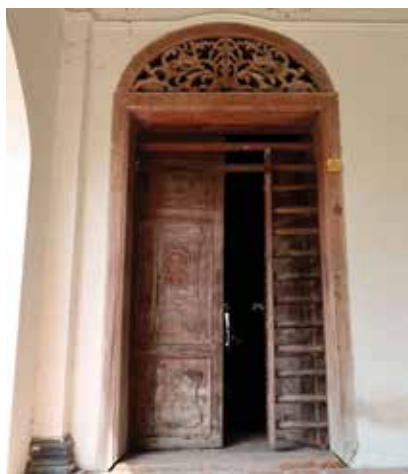
Entrance of Rumah Besar, with carved wooden fanlight above the door and timber security grill, showing the workmanship of Chinese carpenters
