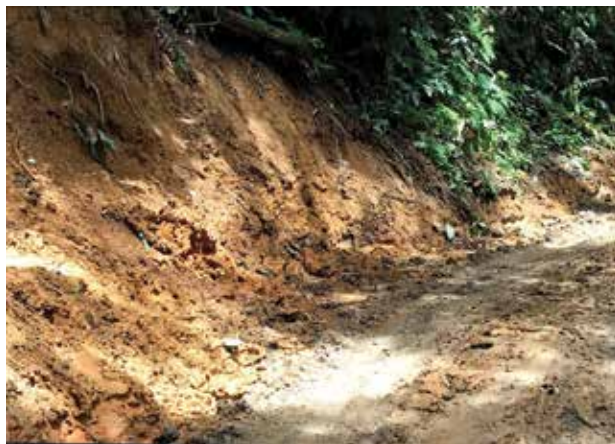
Excavator teeth marks on the damaged slope. This is new damage to the government public road. According to Orang Asli witnesses, the excavator carved out the slope to widen the road, when it was being brought up the mountain. Pic by Roz Hussin.
