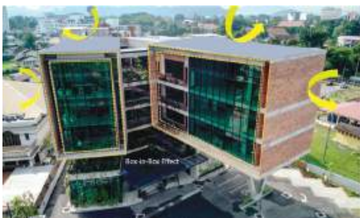
The box-in-a-box effect prevents heat from the east and west from penetrating into the building. When combined with the thick roof insulation, temperatures within the building was kept highly stable.
